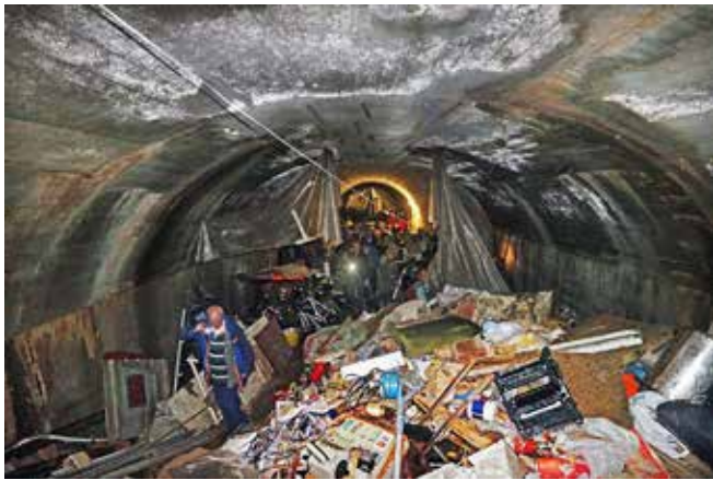
Progressing along the tunnel large quantities of domestic junk have been stored
